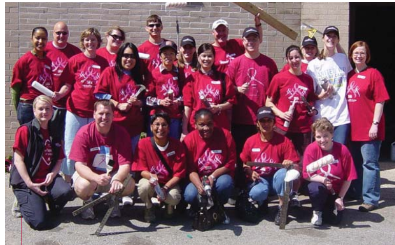
CIBC employees participated in a United Way Day of Caring at the Jane and Finch Boys and Girls Club in northwest Toronto. Volunteers helped in the renovation of "The Garage", an old garage that is being converted into 1,800 square feet of programming space for youth in this neighbourhood.
