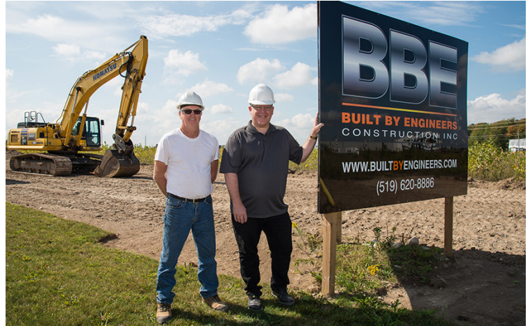
Brian Collier (right), founder of Built by Engineers Construction Inc., and his team, including Roy Case (left), are currently working on a 13,000 square-foot state-of-the-art veterinary clinic in Cambridge. Jon Nicholls Photography
